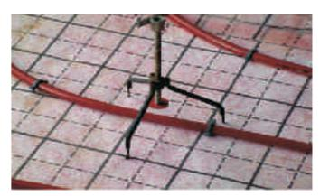
The screed level indicators are laser levelled to the datum prior to pouring.
