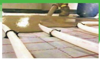
The screed flows around the underfloor heating pipes eliminating air pockets therefore improving heat transmission across the floor. The thickness of Flo-screed for underfloor heating will be 30mm+ the diameter of the pipe. Typically 50mm.
